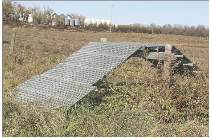
Quad ramp built by Jack to cross fence
