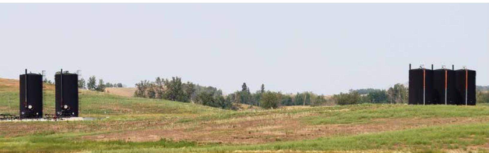
Heavy oil tanks dot the topography in the area
